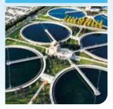
Keeping water clean takes a lot of energy — in fact, up to 3% of all electricity produced. But introduce oxygen into the treatment process and energy use falls while ammonia removal rises. The result? More capacity, less sludge, lower costs.
