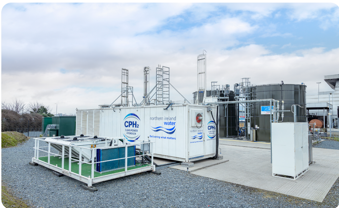
Figure 10: Operational CPH2 electrolyser at Northern Ireland Water, Belfast
