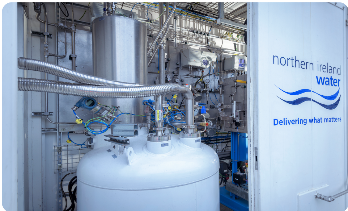
Figure 9: Cryogenic Separator from CPH2 MFE110 on site in Belfast.
